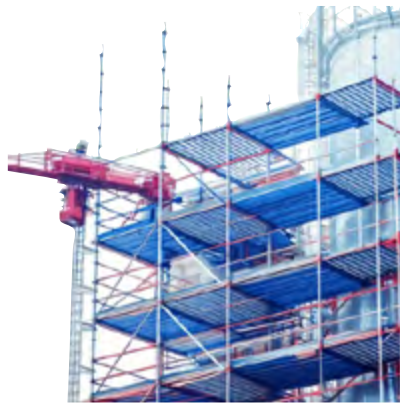
a battery powered lifting bot transports equipment to workers at heights
